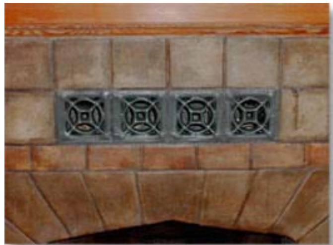
Restored fascia. Job complete.
