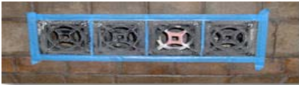
Vent repair in place.
