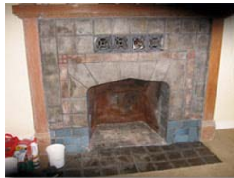
A fireplace in need of repair.
