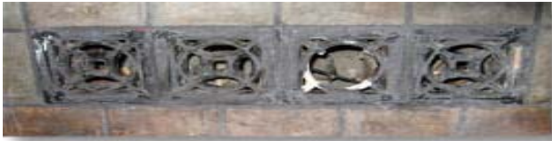
Detail of the vent tiles.
