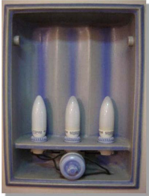
The electric fixture was initially designed for three heating elements that were about twice the height of these light bulbs. Photos courtesy Lou Starr.
