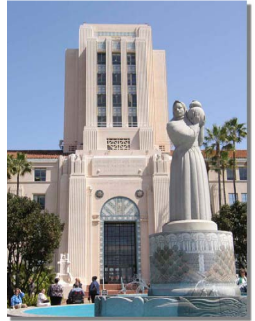
Donal Hord’s “Guardian of the Waters” stands before the San Diego County Administration Building.
