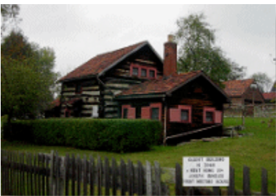
Check out the handmade roof tiles!
