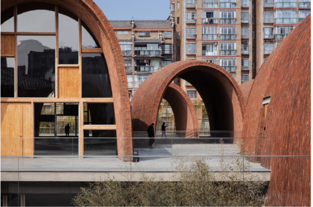
A view of the exterior of the foyer with adjacent open-ended vaults. (Courtesy of schranimage, via v2com)
