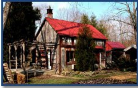
Unison Pottery and Tile Works, Unison Virginia.
