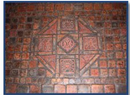
Moravian floor tiles at Grace Church.
